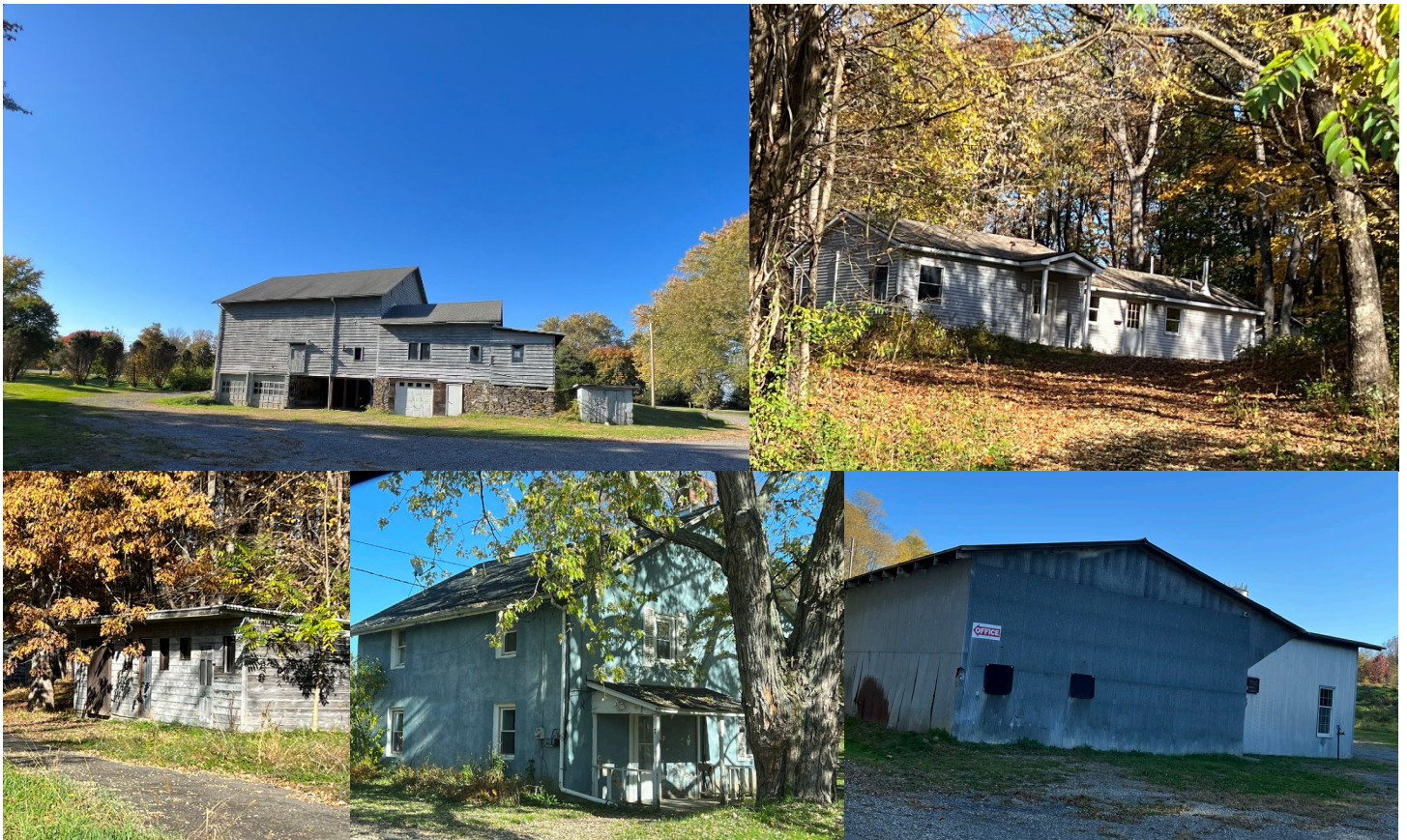
Image 3. Buildings on the Cookingham Farm Property.
